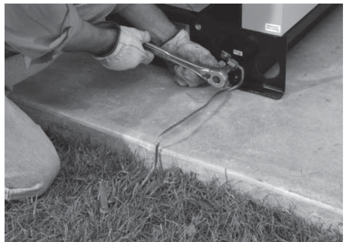
Figure 1.5 — Connect Ground Wire
