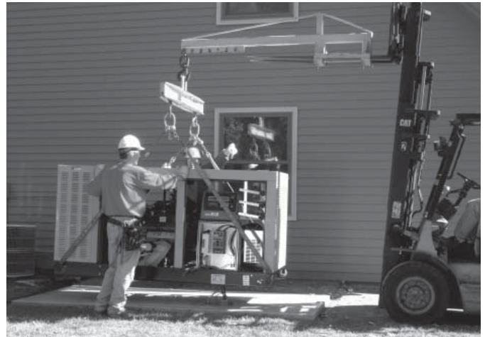
Figure 1.4 — Lifting the Generator
