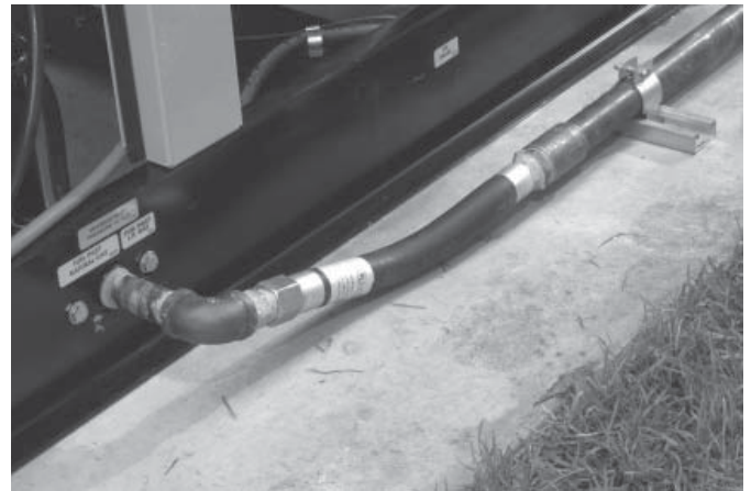
Figure 1.8 — Flexible Fuel Line
