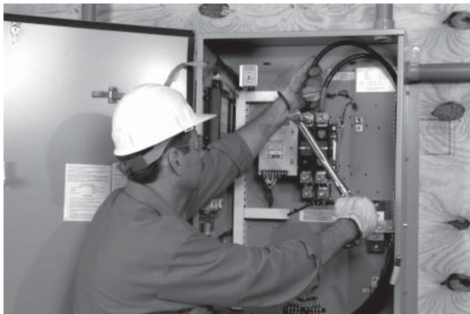
Figure 3.5 — Torque Lugs
