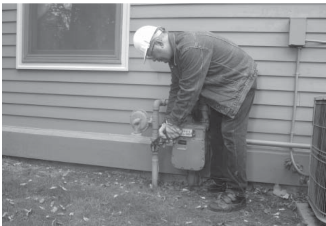
Figure 1.7 — Manual Shutoff Valve
