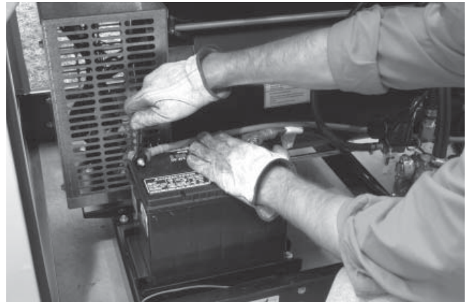
Figure 1.15 — Check Terminal Connections
